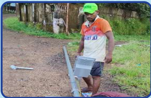
Installation of solar street lights at Attargaon
