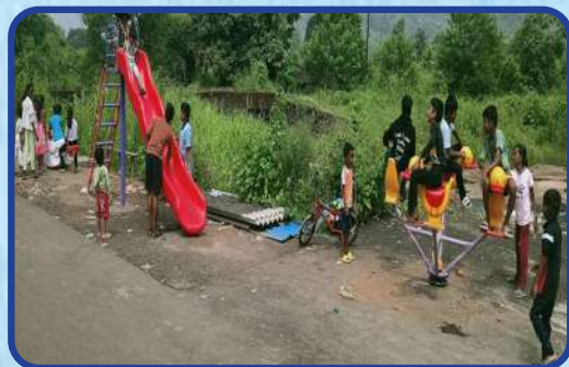
Building playground for children at Beedkhurd
